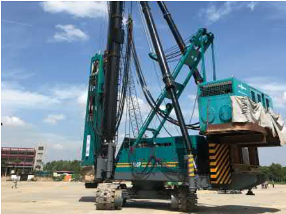
LH130 + HHP14 Commissiong in Hongkong
