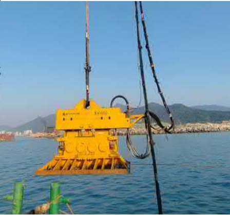
SV400 for under water compaction In Shenzhen, China
