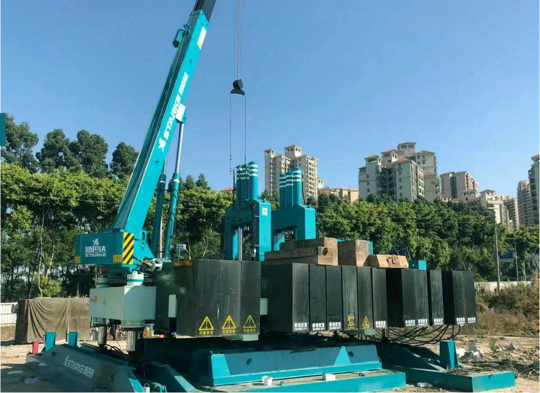
PH900B At Guangzhou construction site
