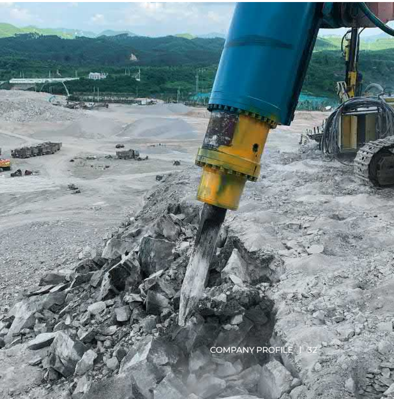
HHR100 Mass rock is broken by high strike energy
