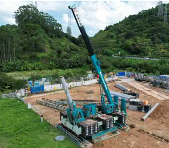
PH350X Piling 30°battered pile near Baiyun airport
