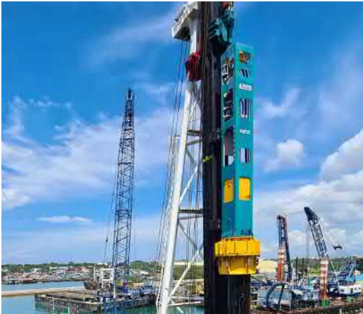
HHP20 for port construction In Malaysia
