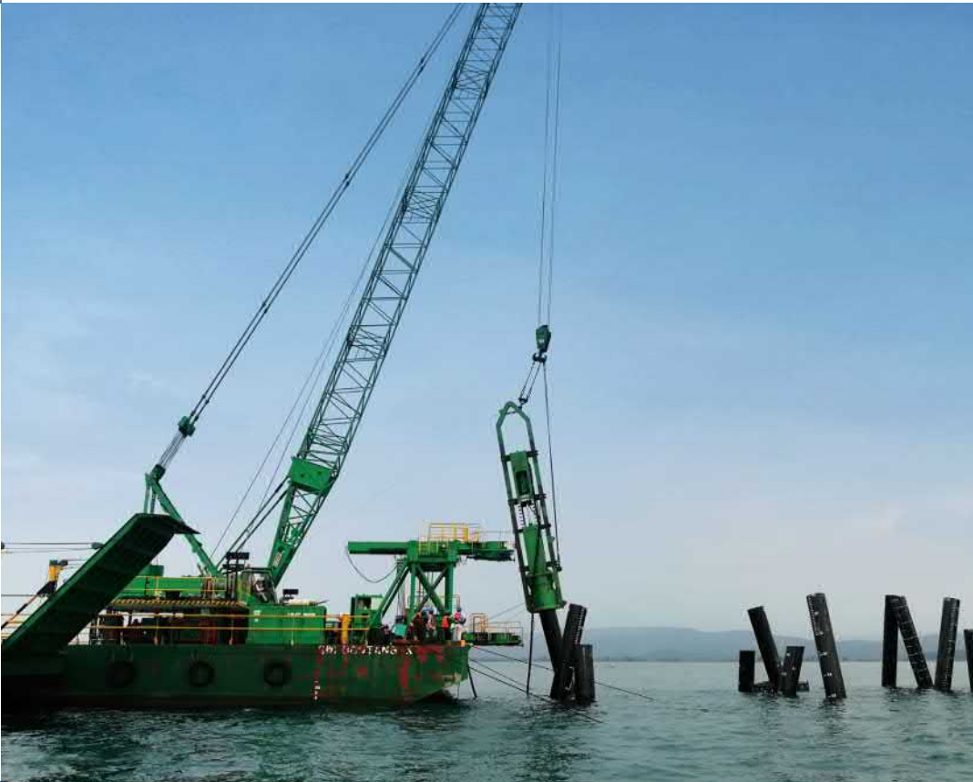
HHP14 for raked pile In Indonesia
