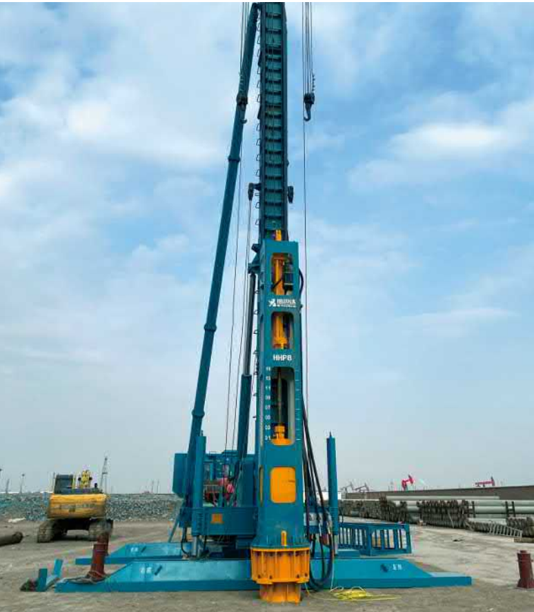
JB62H+HHP8 Port project in Tianjin
