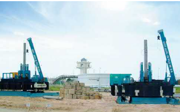
PH600 6 pile drivers at construction site in Malaysia
