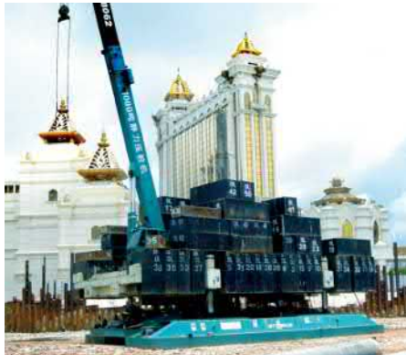
PH1000 construction site at Galaxy Hotel Macau
