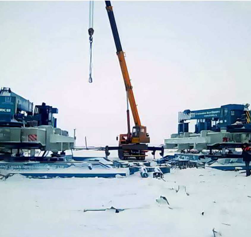
PH320 construction in Russia
