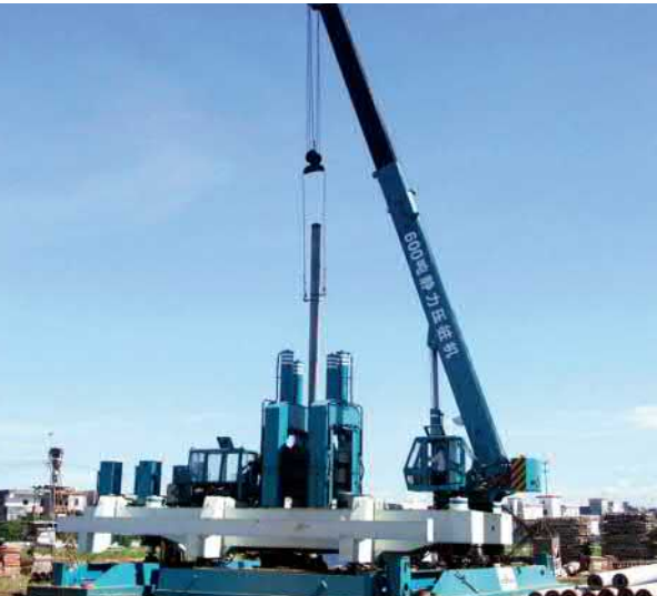
PH600 At China construction site
